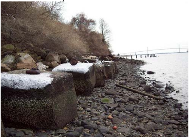
Photo E.6 –View of concrete blocks used for anchoring ships. Note: About 15 of these blocks were noted and spanned roughly 80 feet. The blocks measured approximately 6x6x4 feet in size.
