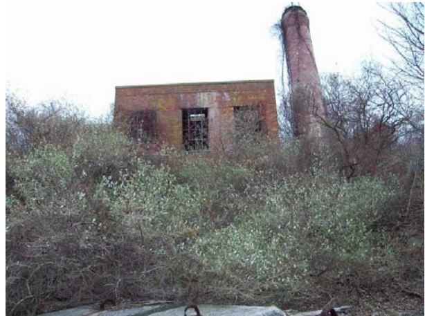
Photo E.14 – View of the incinerator building located adjacent to (north of) the Disposal Area (MRS 1).
