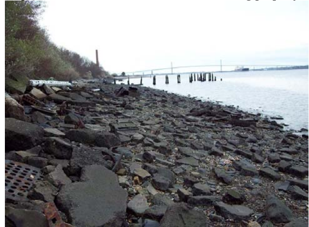
Photo E.4 – View looking south towards the small pier from MRS 1 (Disposal Area). Note: The beach area was cluttered with various metal debris, concrete, building materials and tar deposits.
