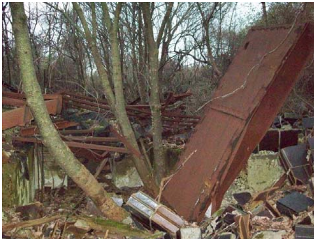
Photo E.23 – View of former Bunker 11 (now collapsed) in PAOI 1. Note: The bunker had completely collapsed and conditions were unsafe to enter.
