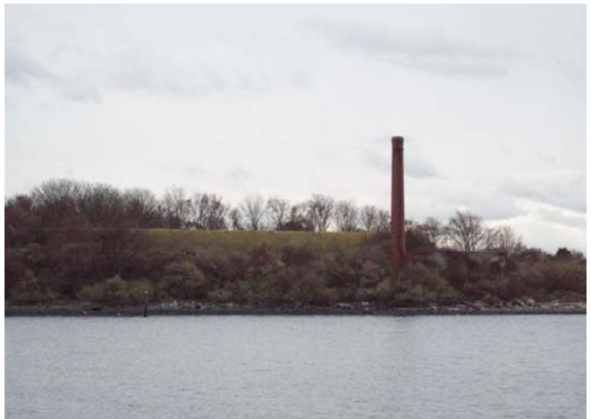
Photo E.24 –View of the Torpedo Store House (PAOI 2) approaching Gould Island.
