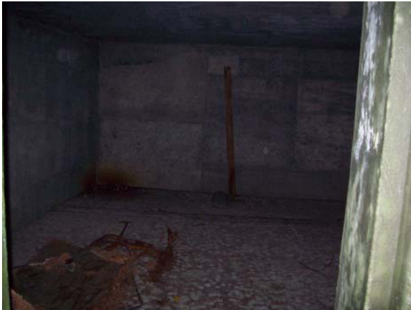
Photo E.27 – View of the aforementioned bunker in Photograph E-19 (PAOI 3). The floor at the entrance of the bunker was covered in leaves however the inside of the bunker had a bare concrete floor and there were no evidence of drains however cultural debris was noted on the floor.
